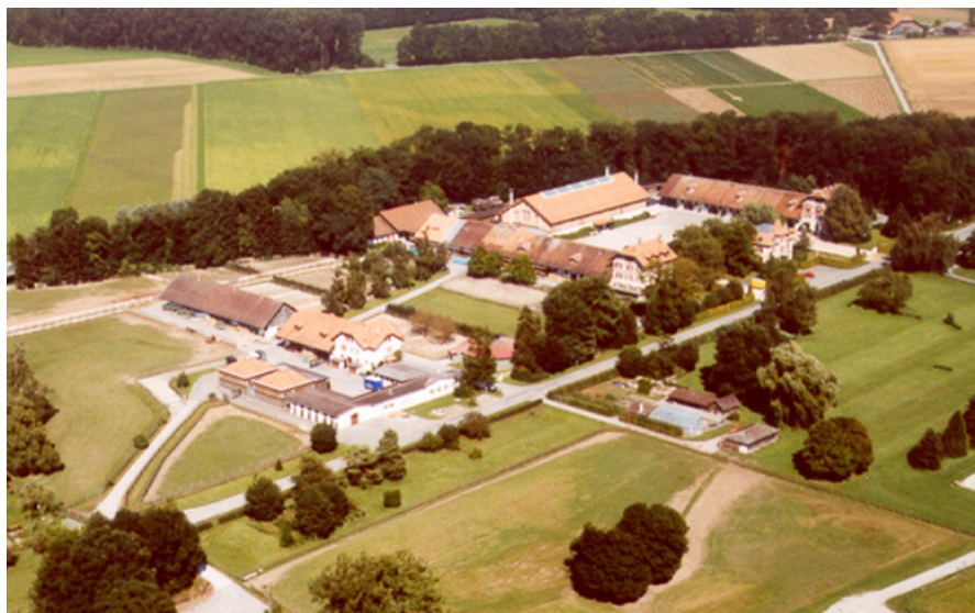
Avenches: Contemporary aerial view of the stud farm with horse clinic
