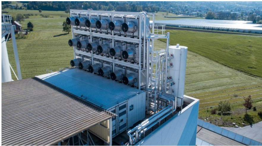
Figure 11. Climeworks' commercial DAC plant annually delivering about 900 tonnes of food-grade CO 2 as fertiliser to a greenhouse operated by Gebrüder Meier in the town of Hinwil (Canton of Zurich). A nearby waste-to-energy plant supplies the heat to regenerate the proprietary capture material. 76
