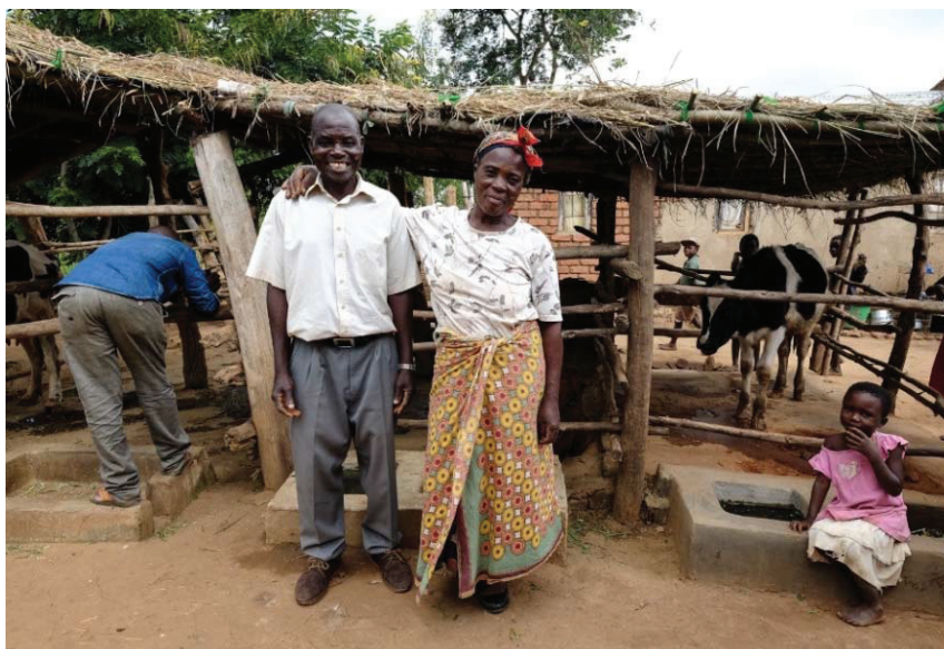
Photo 7b: Prevention of mastitis has improved significantly as a result. Cleaning of the floor has also become much easier.
