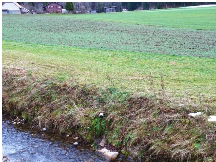
Figure 5: A drain discharging into a small watercourse in Rueti, Canton Bern (photo: Urs Schönenberger).
