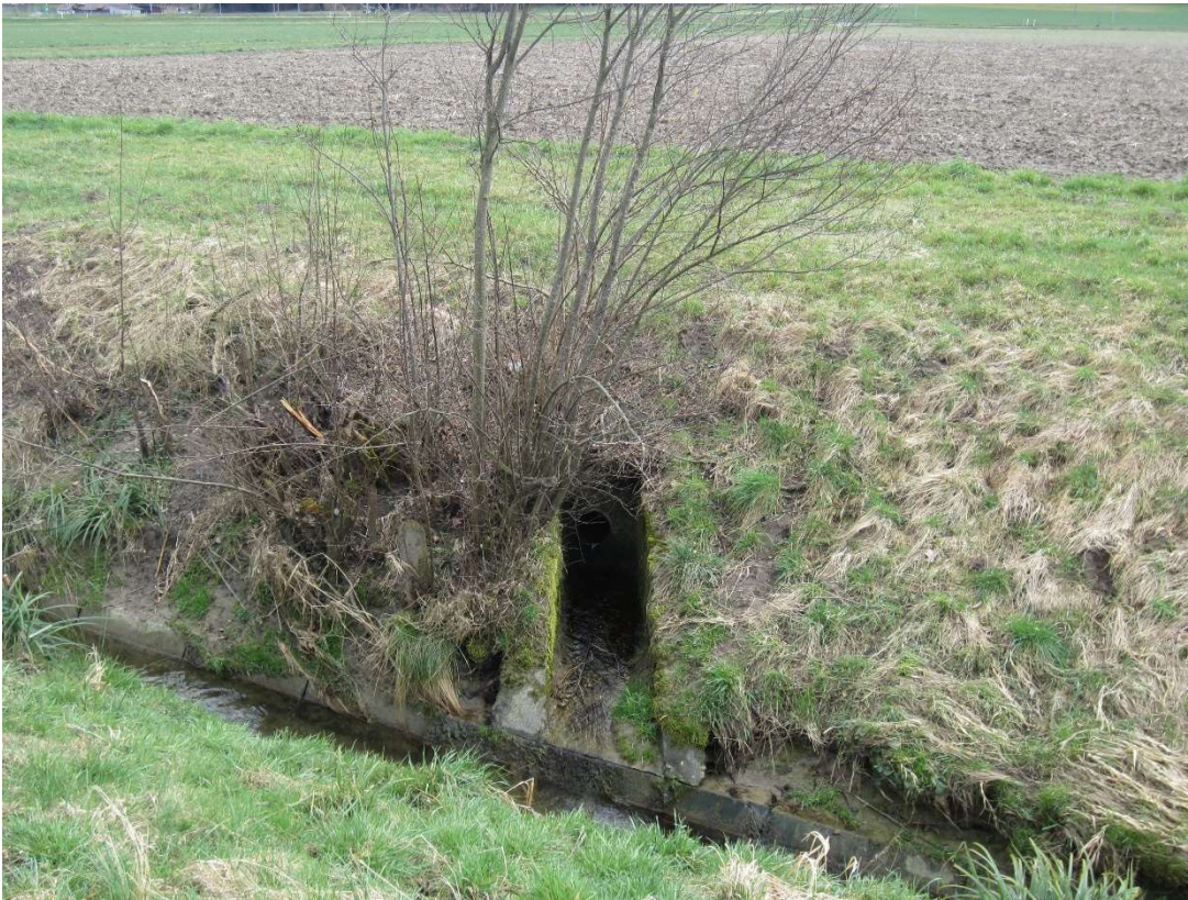
Figure 2: A drain discharging into a canalized small watercourse.
